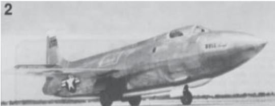
*Image 2: Bell X-1D had short career, just one flight. On July 24, 1951, its nose gear failed during landing.*
